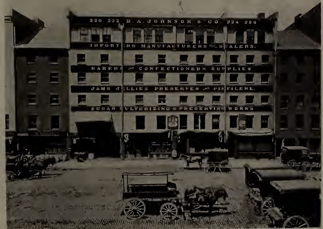
BUILDING OCCUPIED BY H. A. JOHNSON & CO., 222 and 224 State Street.
